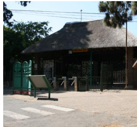
Upper Park Drive entrance - currently under construction to expand parking facilities.
