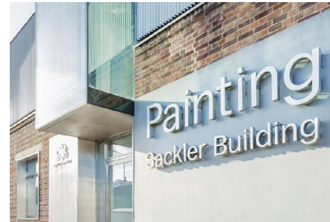
Fig 99, Entrance showing original masonry and new roof structure junction
