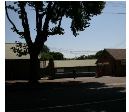
Service entrance on Upper Park Drive
