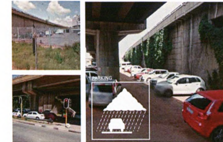
SIMMONS STREET UNDERPASS
