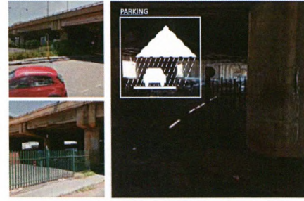
LOVEDAY ROAD UNDERPASS
