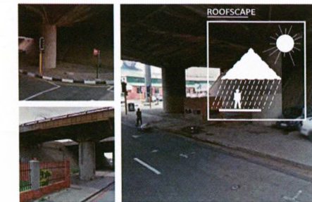
USSHER STREET UNDERPASS
