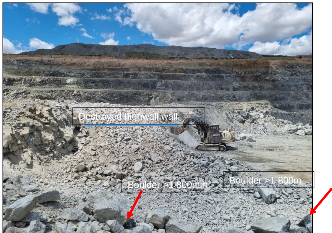
Figure 8.1 Blasted muck pile boulders and destroyed high wall.
