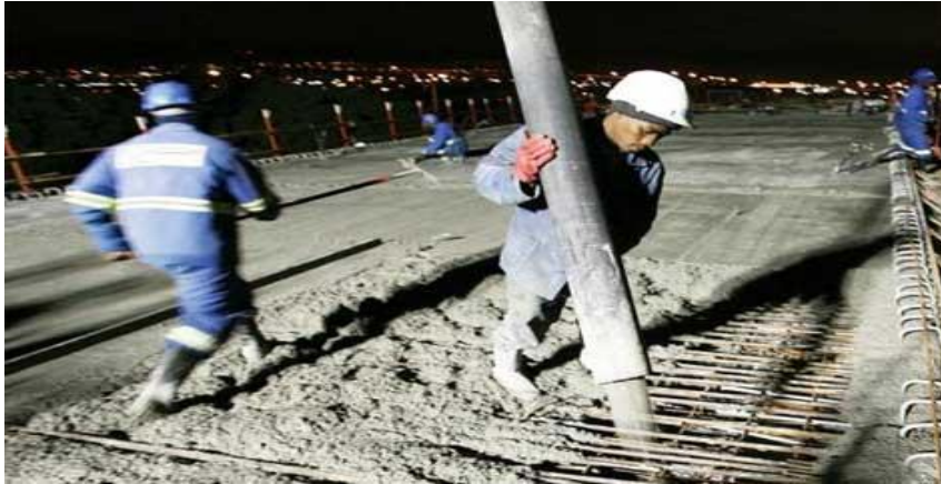
Figure 2.2: Concrete paving construction at night
