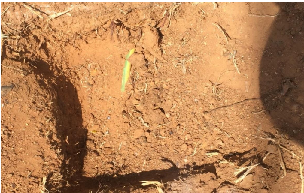
Figure 4.3: Electrical cables exposed at pole no. JGC 106/3/14 during sampling collection (Rampjapedi, 2015)
