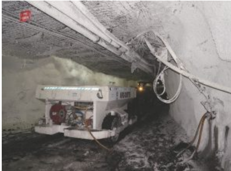
Figure 4.5: Stone dust applied to a roadway
