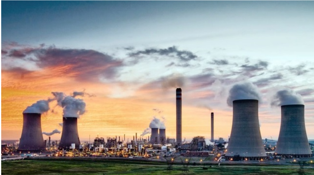
Figure 1.6: The Sasol Secunda Synfuels Operations, Mpumalanga, South Africa (IOL, 2019)
