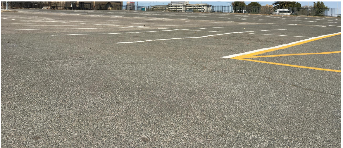
Figure 3.5: Tarmac road condition used for testing.
