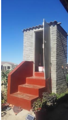
Fig 5.3 Sky Loo Toilet used in Victoria Ranch (Source: Author's Own Photograph, August 2016)
