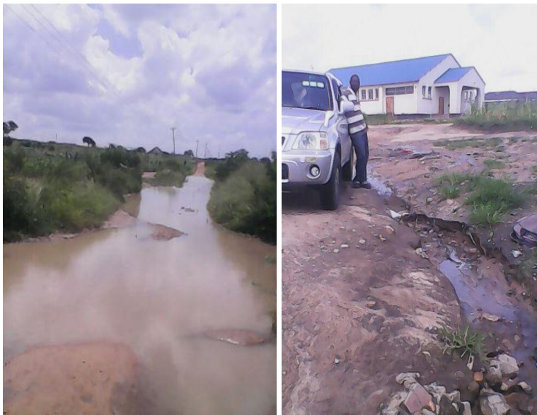
Fig 5.2 Stagnant water in a road due to poor drainage(left) Eroded road due to rainfall(right)
