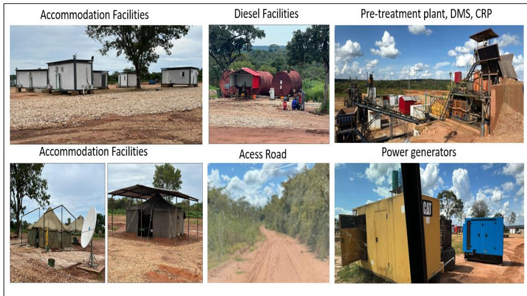
Figure 4.6 Infrastructure at Project A
