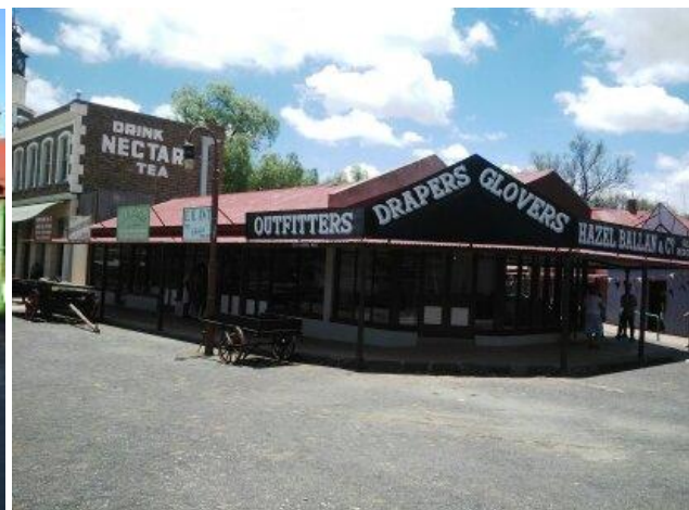
Figure 5: Some structure of the Old Town
