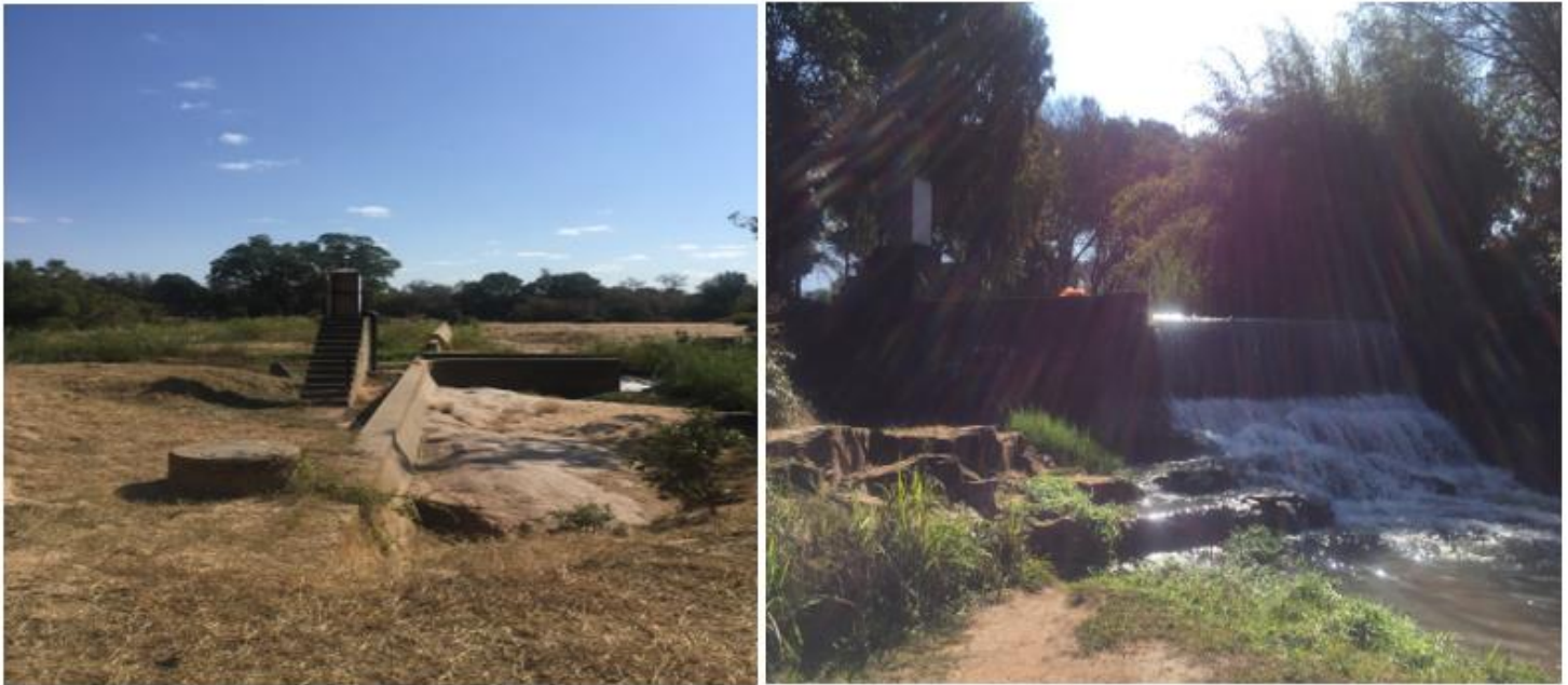
Figure 6: A weir is a flow measurement structure that spans across the width of a river—it consists of a low impoundment which has a flow gauging section and a data capture house/hart located in the highest flood level. In this image is an example of South African rivers weir station design—at observation stations X3H008 on the left and X3H002 on the right.
