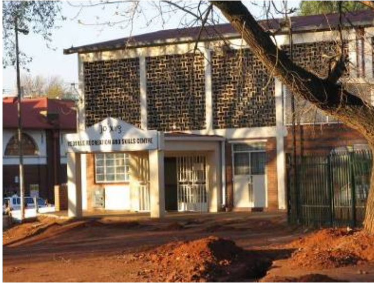
Figure 9: Yeoville Park and Recreation Centre dug up and abandoned (2006).
