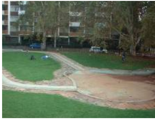
Figure 11: Derelict Water Feature on Southern end of Park (2004).
