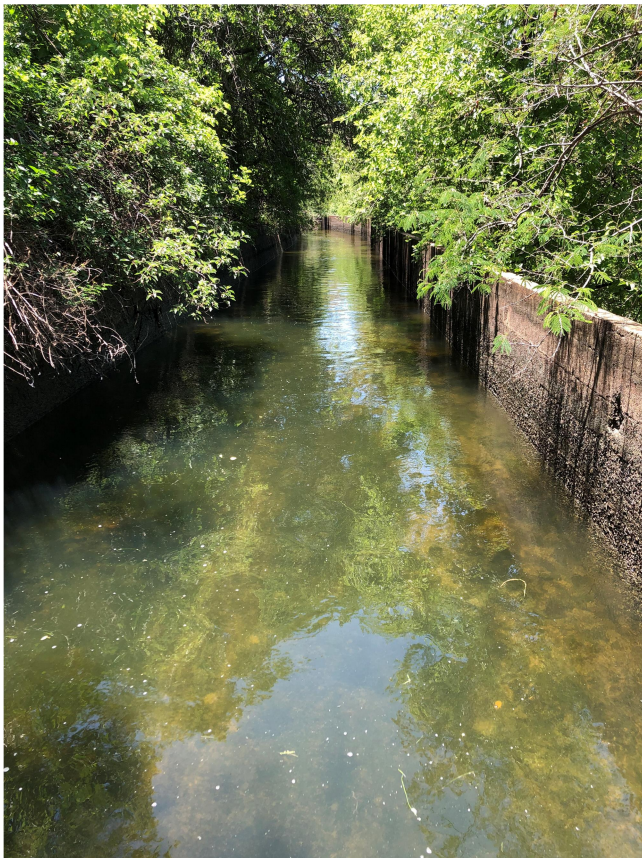
Fig. 3.2.1 (e): Photograph of right canal from above.
