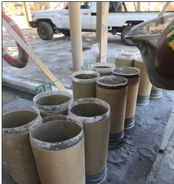
Figure 3-3: Backfill slurry cast into cylindrical moulds
