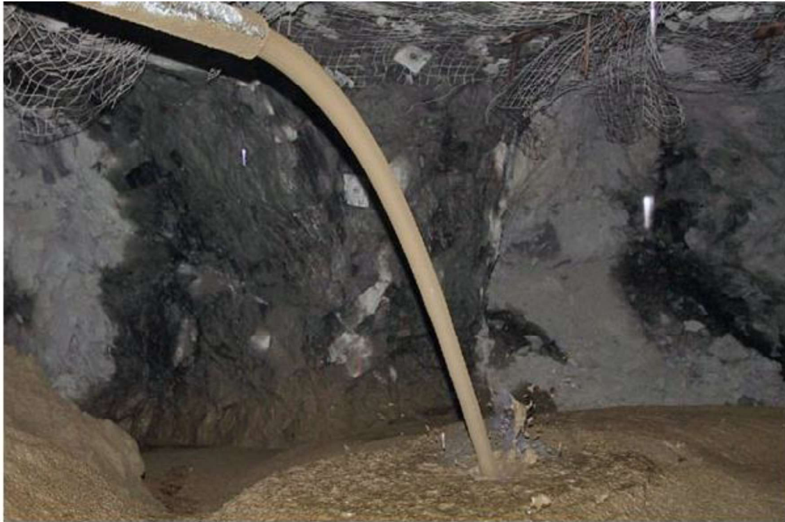
Figure 1-1: Filling an underground stope using hydraulic fill (Barrick Gold, 2020)
