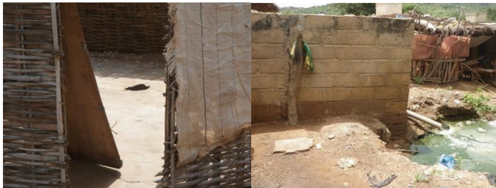
Figure 1.4. Examples of pit toilet construction in Madine village
