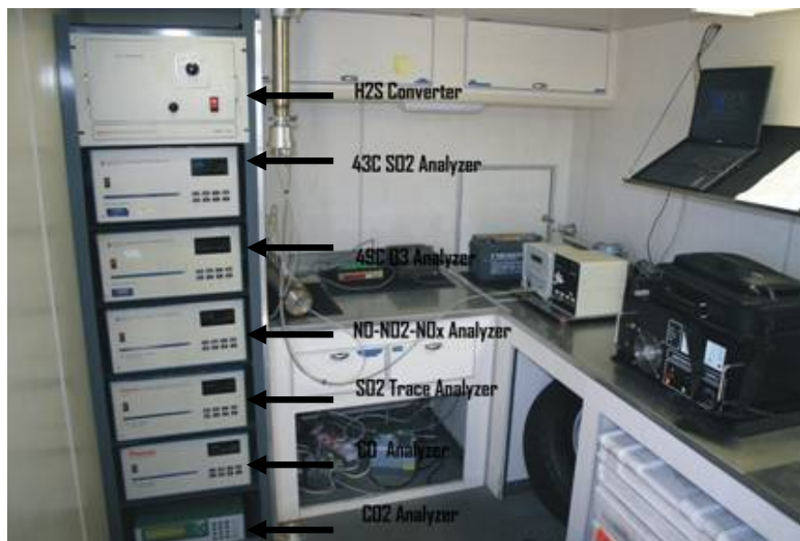
Figure 3.5: Ambient gas analysers housed in the mobile monitoring station
