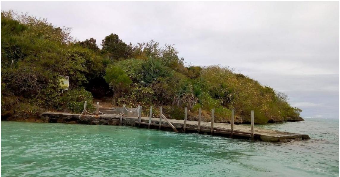
Figure 4.4: The entrance of IAA with the jetty. A photo (GG002-10) captured from the boat by Shreena
