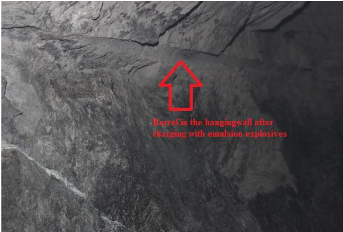
Figure 6.16: Visible barrels after charging with emulsion
