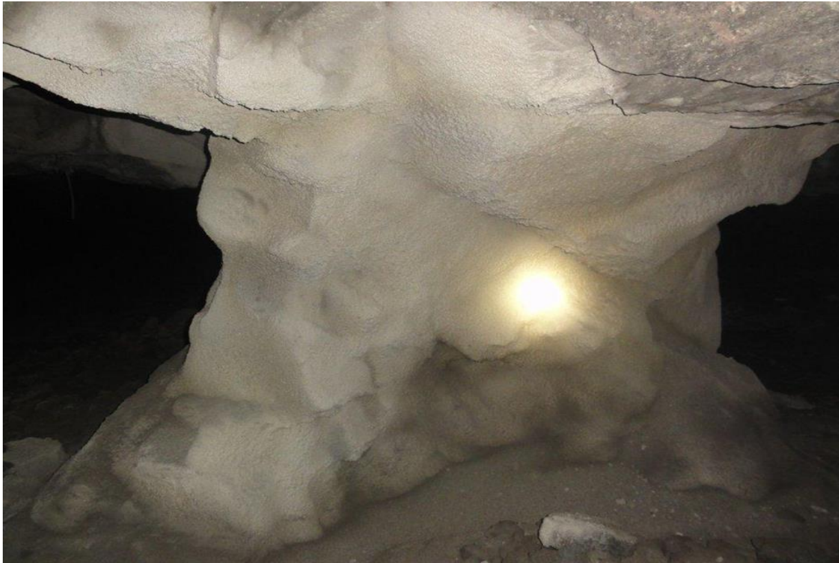
Figure 5.5: Shotcreted pillar at case study mine
