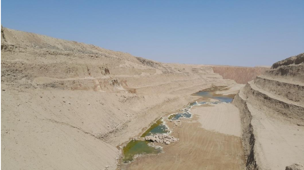
Figure 29. The currently ongoing seepage at Langerheinrich mine from the lined new tailing dumps
