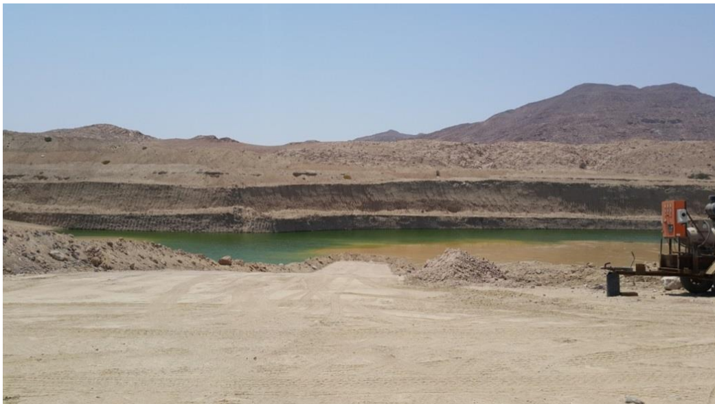
Figure 30. The ponding of water on the new tailings dumps
