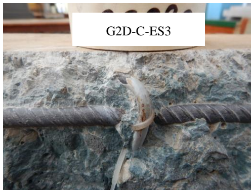
Figure E. 5: Photographs of corroded reinforcement bars in cracked PC/SL concrete.
