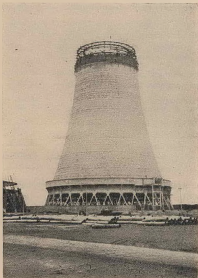
11. General view showing the shell nearing completion.
