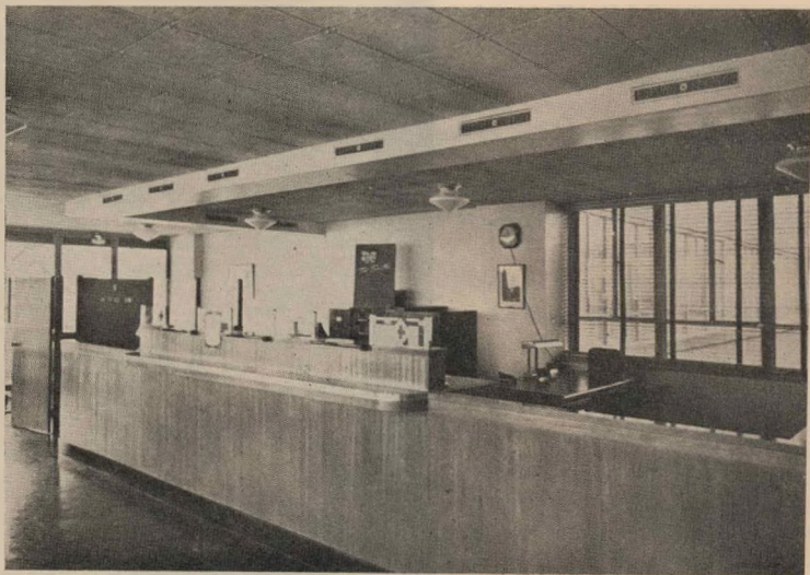
ABOVE: One of the upper-level sidewalks which are concrete cantilevered extensions of the floor slabs. Adjacent walls of the offices are of glazed panels and doors. BELOW: Typical office space. Partitions may be placed at any point; access to utilities, installed between furred ceilings and floor-slab construction, is by means of removable squares of acoustic material with which the ceiling is surfaced.
