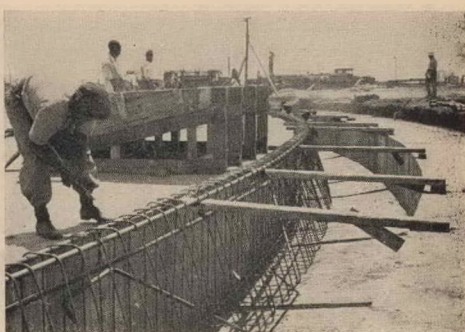
5. Detail of the steel reinforcement of the great ring beam.
