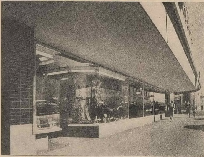
Street level view of the shops, protected by the reinforced concrete cantilevered canopy.
