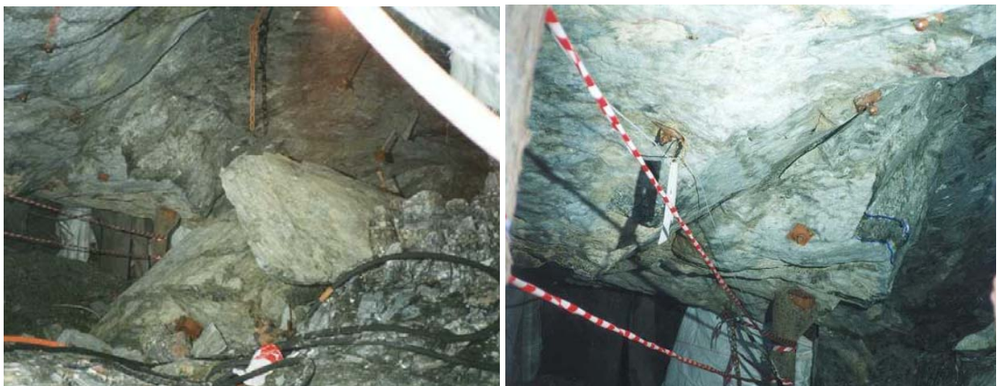
Figure 1.3 Dome collapse with part of the dome still intact in the hangingwall
