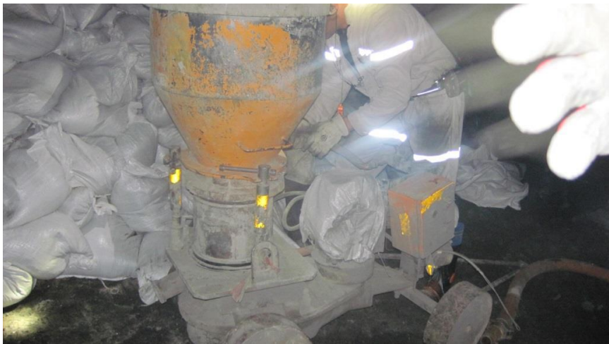
Figure A- 10: Bulk shotcrete material
