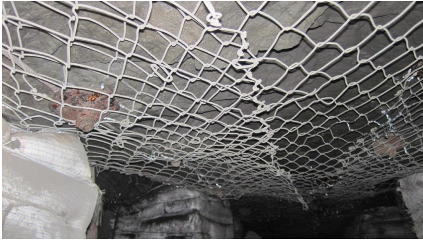
Figure A- 22: Ultra-strength chain link mesh installation
