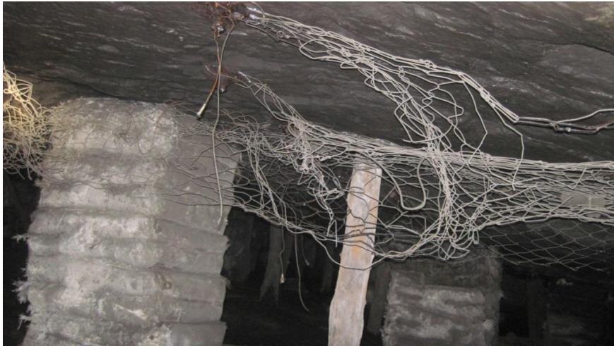
Figure A- 23: Scraper damage on chain link
