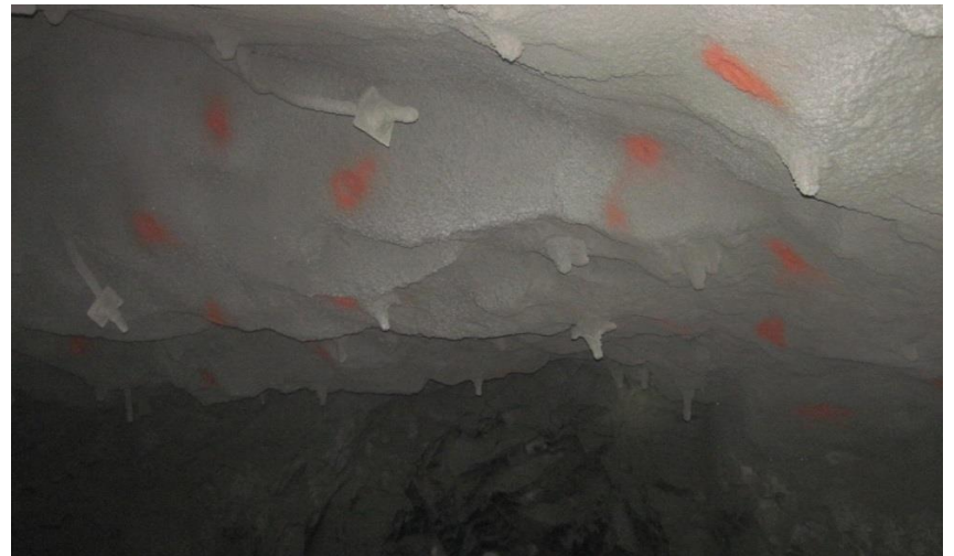
Figure A- 12: Dyke condition after shotcreting
