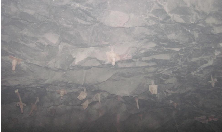
Figure A- 9: Dyke conditions to be shotcreted
