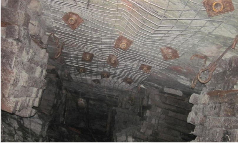
Figure A- 16: Good weld mesh condition in a gully
