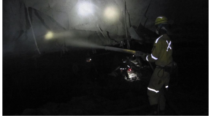
Figure A- 11: Shotcrete application procedure
