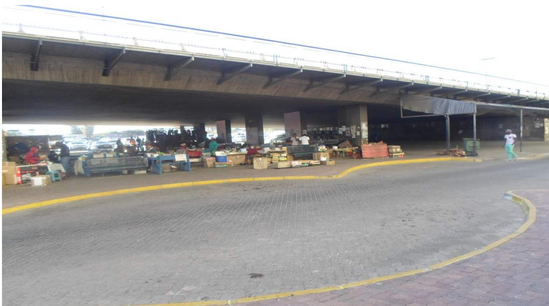
Photo No. 14: Marketplace under the Bridge (before an upgrade)
