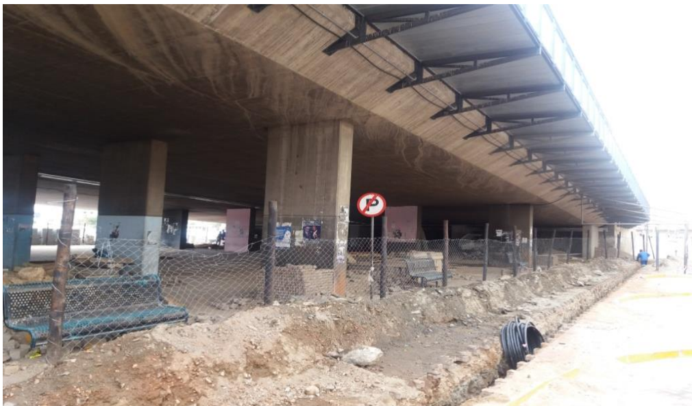
Photo No. 15: Wernhil Market Upgrade Underway 538
