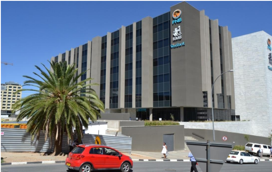
Photo 19: FNB New Headquarters 568
