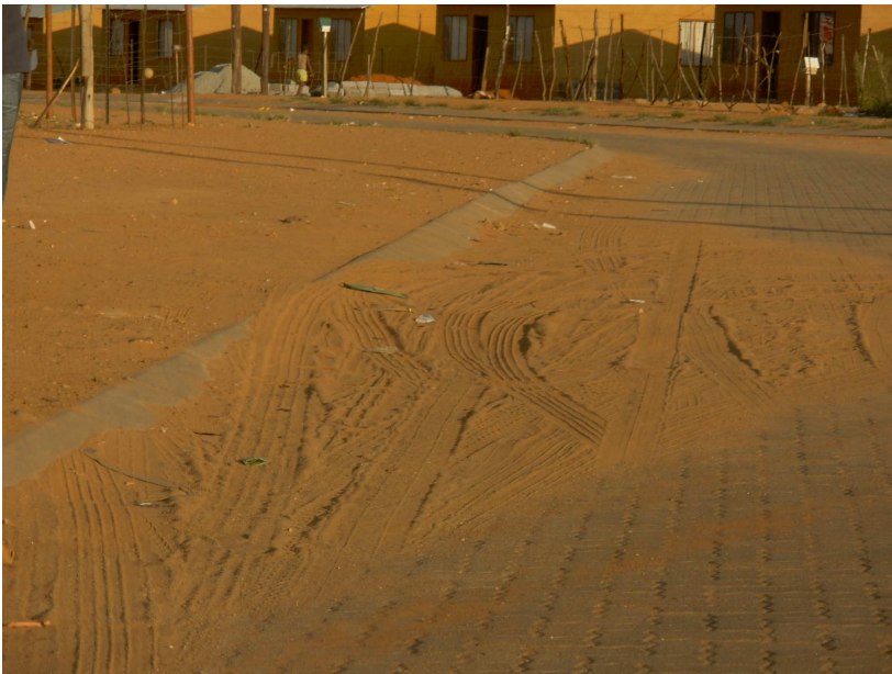
Photograph 4 -: Sandy Road embankments
