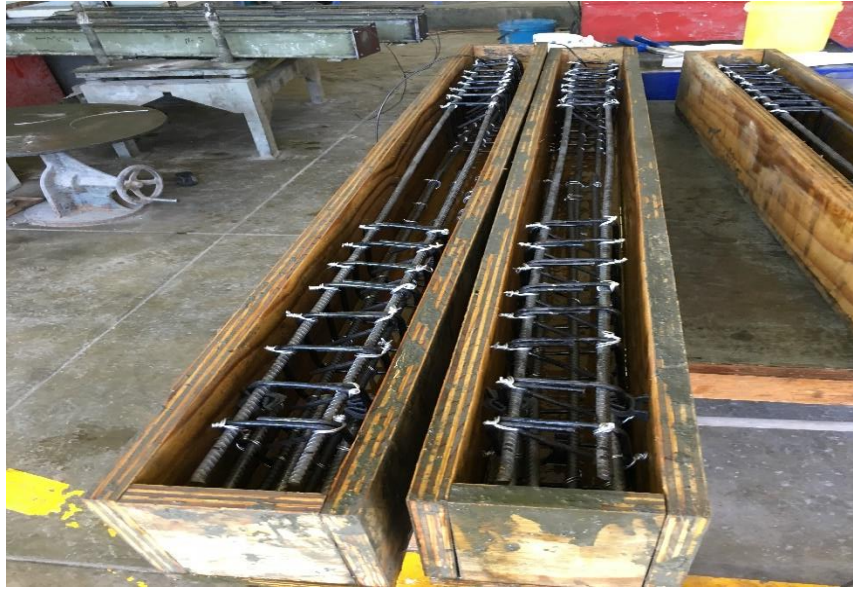
Figure 3. 2: Photograph of moulds prior to concrete casting
