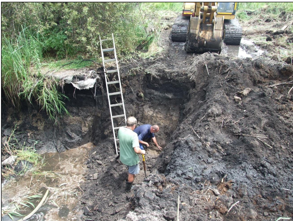
Fig. 4-2: Excavation of Pit C in order to expose a clean vertical stratigraphic face for OSL sampling.
