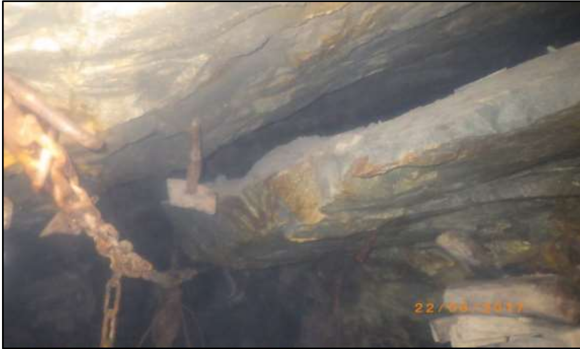
Figure 4.27 Convergence in advance strike gully (Doornkop Shaft, 2017)
