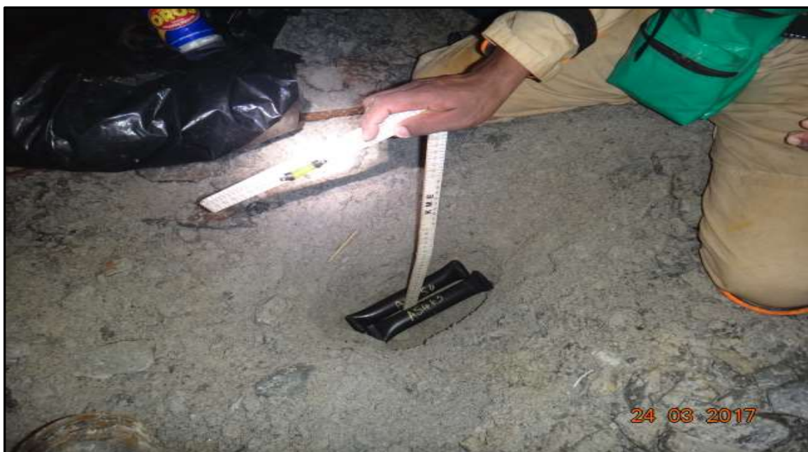
Figure 3.1 Burying of RFID tags in the advance strike gully (Doornkop Shaft, 2017)
