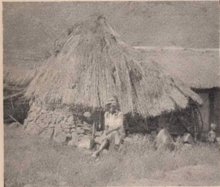
11. "Rondavel" type with stone wall
