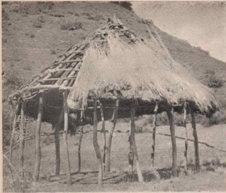
9. Framework of "rondavel" type with circle of posts. Owami
