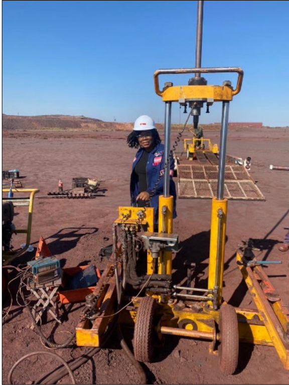
Figure 7. CPTu Rig AT Khumani mine TSF June 2022.
