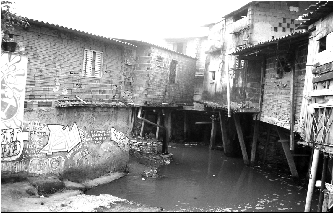
Figure 4.4- Dwellings in favela São Remo , Butanta Sub-municipality, São Paulo. People built their huts over an open sewer from a nearby factory. Photographed by author, February 2005.
