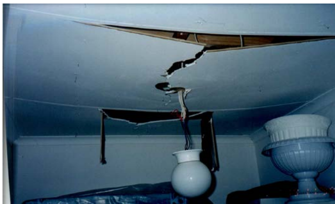
Figure 2.4: Signs of a roof having collapsed. Structural damage caused to a club house building as a result of direct lightning strike (McKechnie and Jandrell, 2008).
