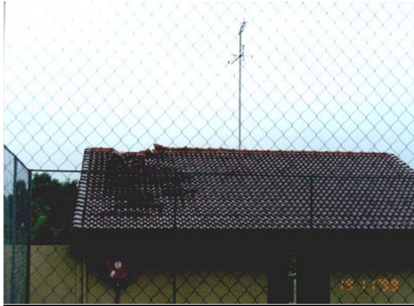
Figure 2.3: Structural damage to a club house due to direct lightning strike (McKechnie and Jandrell, 2008).
