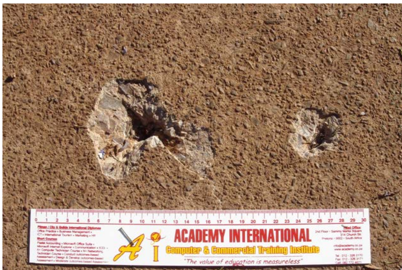
Figure 3.3: Blast / explosion effects from the lightning noted on the concrete pavement on the right side of the victim.
