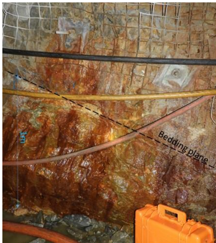
Figure 5-7: Seepage water collected from bedding plane/reef contact at SD 4 and SD5 at SDGM.
