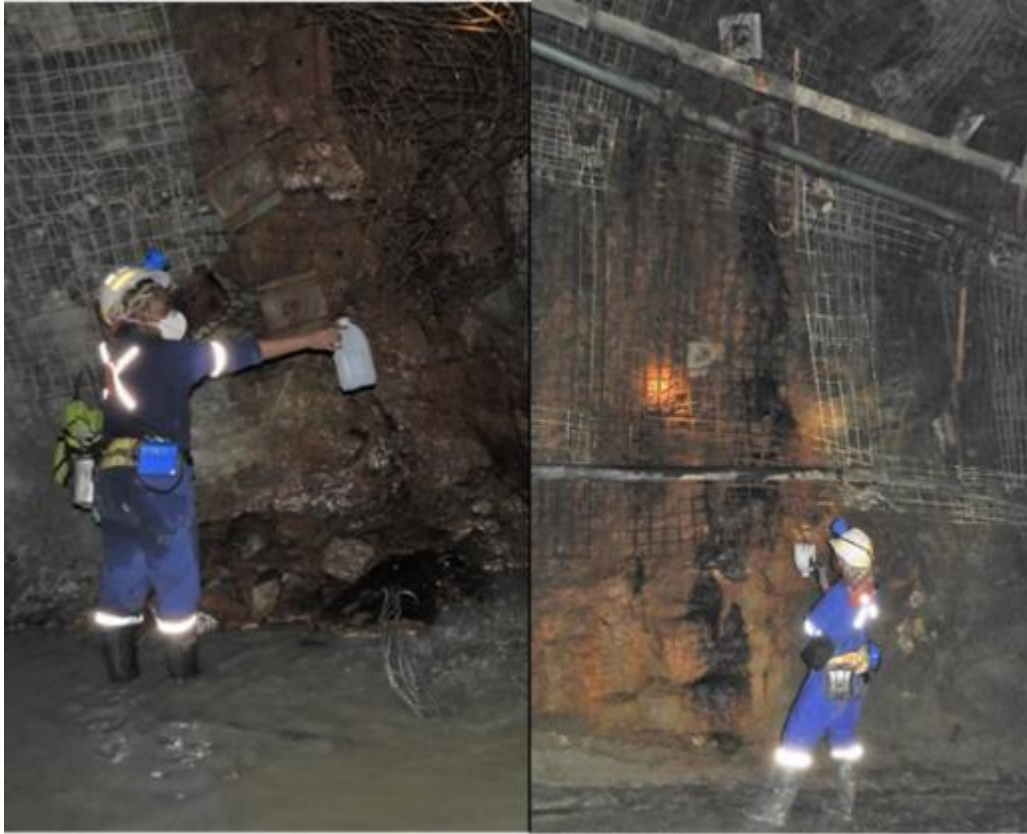
Figure 5-8: Seepage water collection from hanging wall at SDGM associated with mapped faults and joints.
