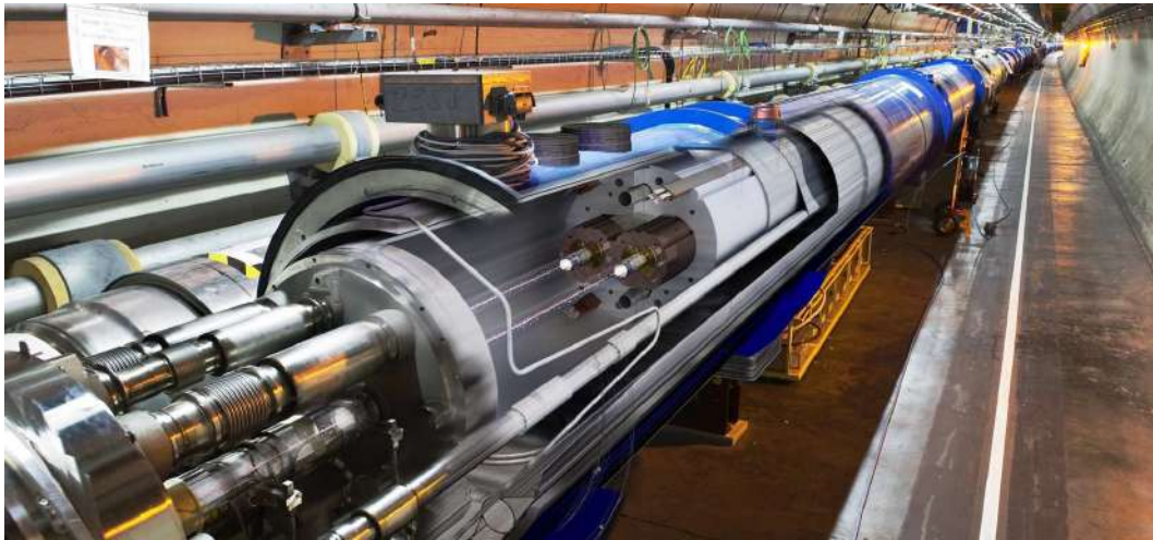
FIGURE 1.2: Inside view of the LHC tunnel [6]
