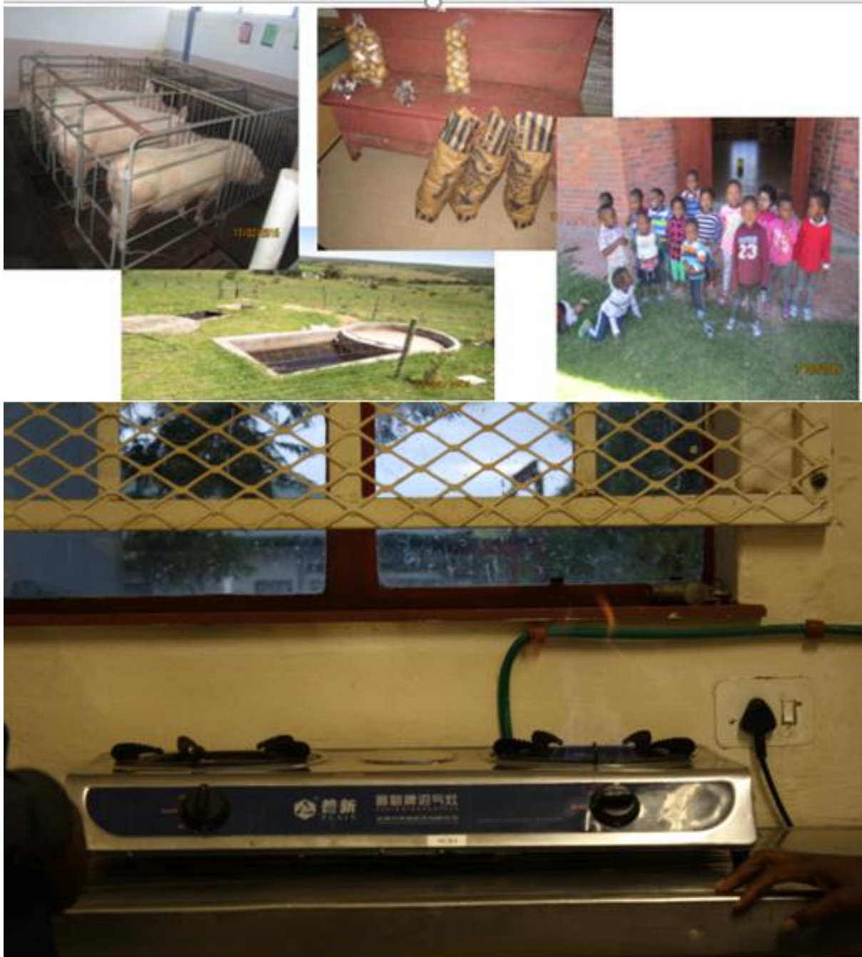
Figure 31: Micro-scale digester cycle – biogas stove from a 12m 3 fixed dome biogas digester installed in Melani (Eastern Cape) Village early childhood development centre.
