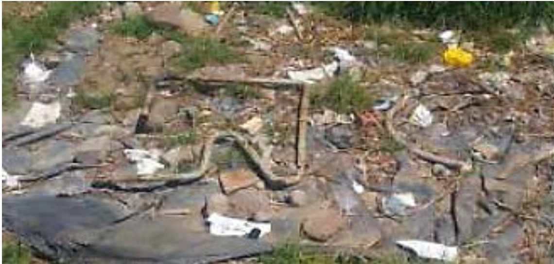
Figure 15: Ballon bag digester damaged in Cedarville (Kwazulu Natal)
