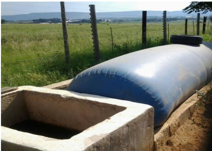
Figure 7: Balloon biodigester plant
