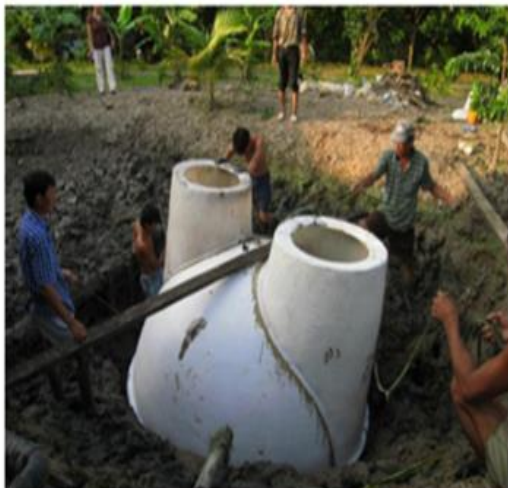
Figure 30: (Left) Biodigester installation in Vietnam
