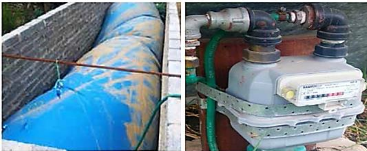
Figure 14: Balloon digester bag in Melani village (Eastern Cape & gas flow meter Source: GIZ (2016).
