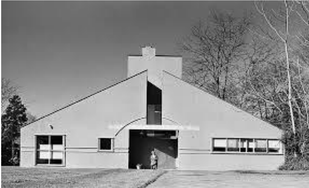
Figure 2-4 Vanna Venturi House located in Chestnut Hill, Pennsylvania built in 1964
