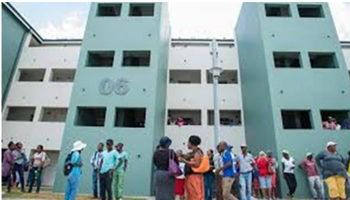
a) Multistorey walk-ups at the Riverside Housing Development
