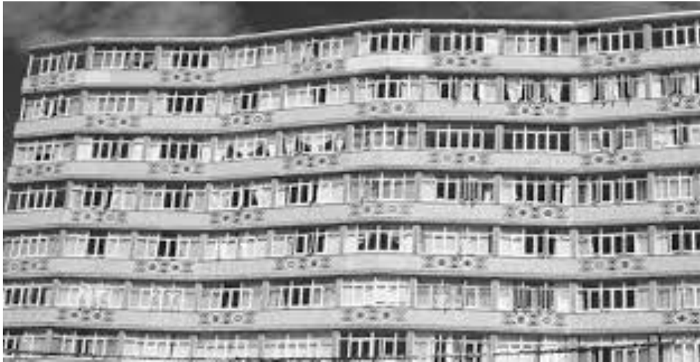
Figure 2-1 Bel Aire flats located along Durban's north beach designed by Reg Buck in 1956
