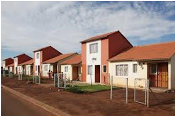
b) Row housing typology at Lufhereng Housing Development
