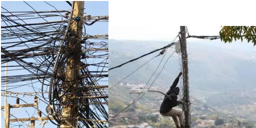
Figure 2.1 (Evans, 2015) and Figure 2. 2 (Peters, 2015): Ways in which the inhabitants of informal settlements steal the electricity.
