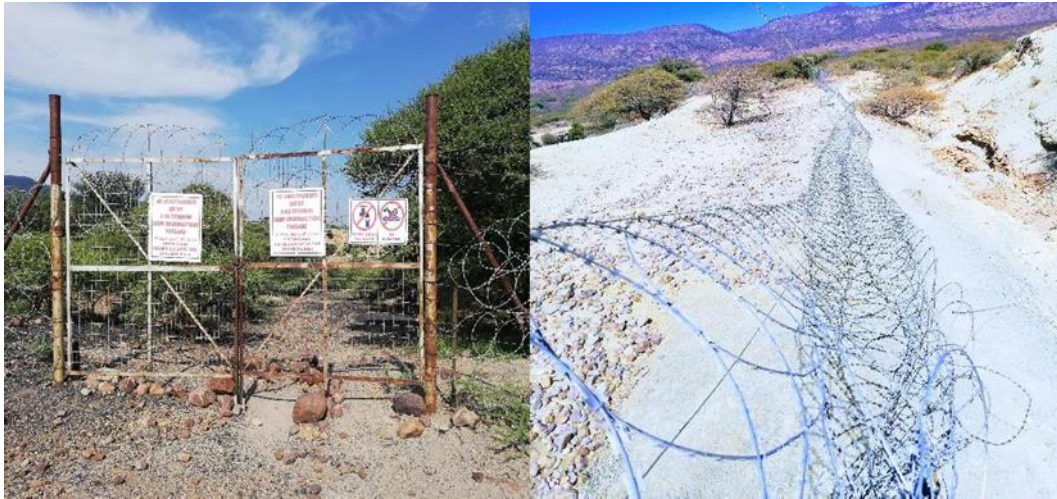
Figure 29: Demarcation fence at the old mine
