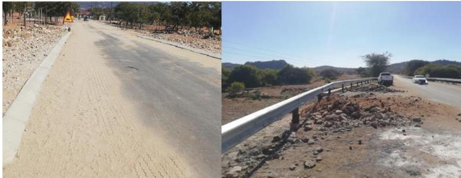
Figure 14: Tar road at Mudimeli Village
