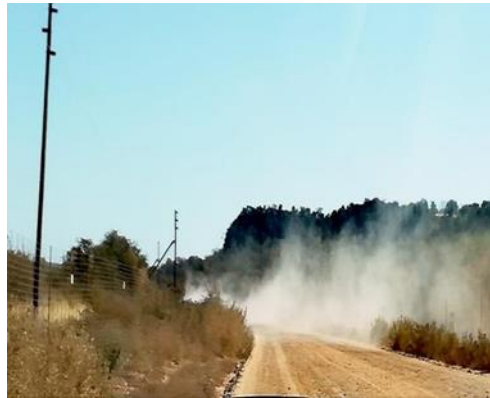
Figure 15: Gravel road from Mudimeli Village to N1
