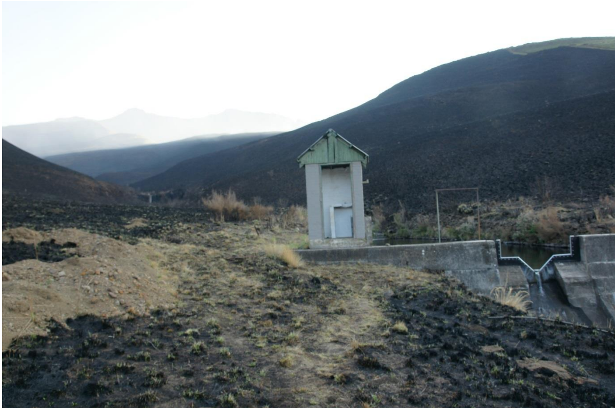
Figure 45 CP04 after it had recently been burned in 2015/09.
