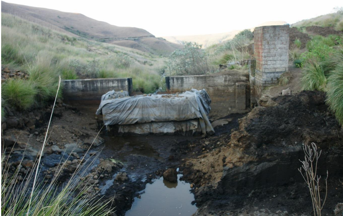
Figure 46 CP03 during the time the weir was being worked on.
