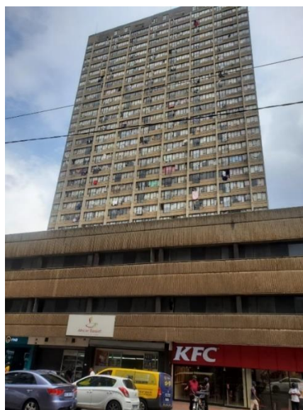
Figure 25: Picture showing a hijacked building with tenants living in it
