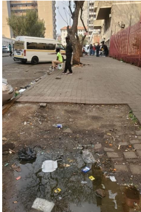
Figure 37: Picture showing a street with unmanaged buildings
