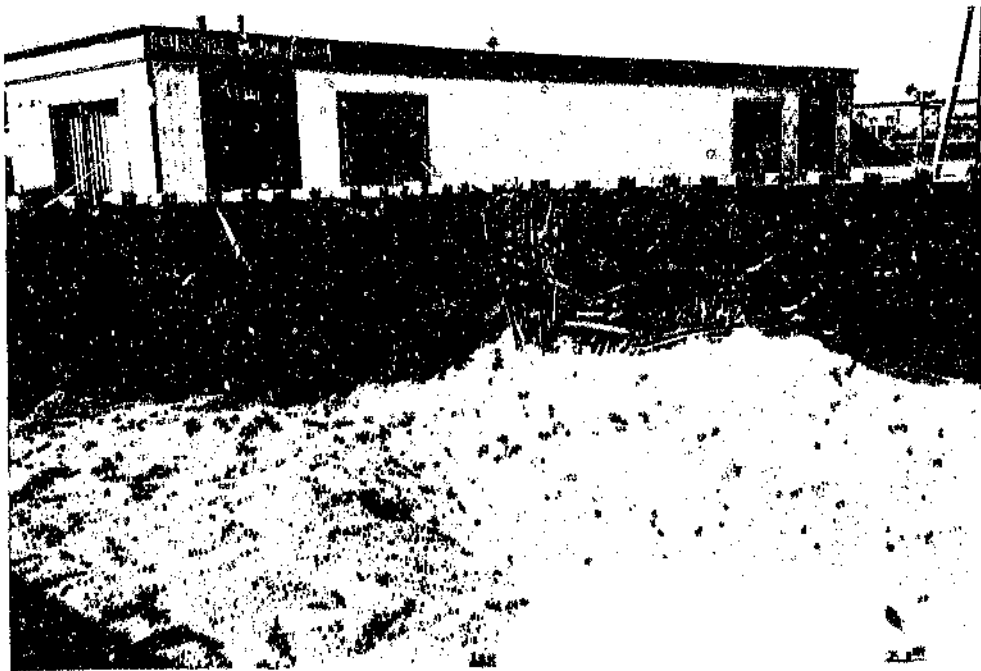
Figure 5.4 Sand Layer Placement
