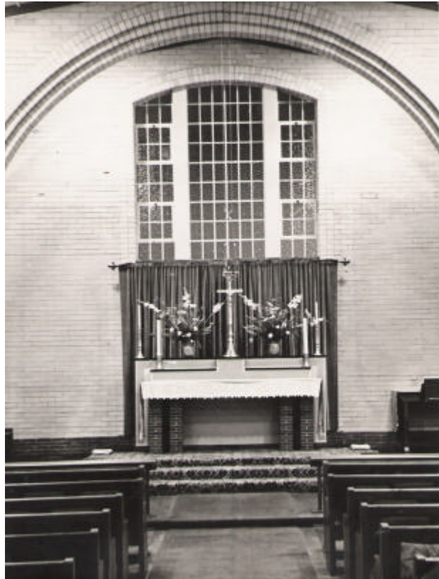
St Thomas' Church The original altar at the West End - 1955
