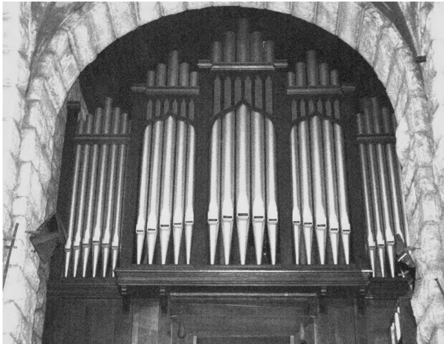
St Boniface Church The organ pipes above the console in the organ loft
