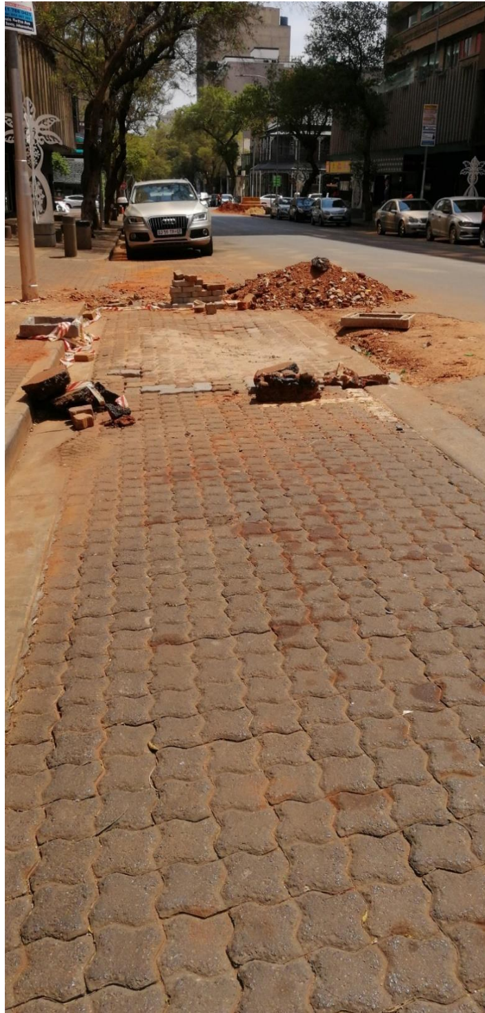
Figure 23: A part of the road that was dug up by Johannesburg Water in Braam. As it has been discussed, the lockdown had impacted the number of staff on the ground deployed by different MoE's and as a result led to instances such as the image where reinstatements could not be done timeously. The BID manager was unimpressed at how this was left and expects them to come to fix this. Image was taken by Rorisang Sojane (2021)
