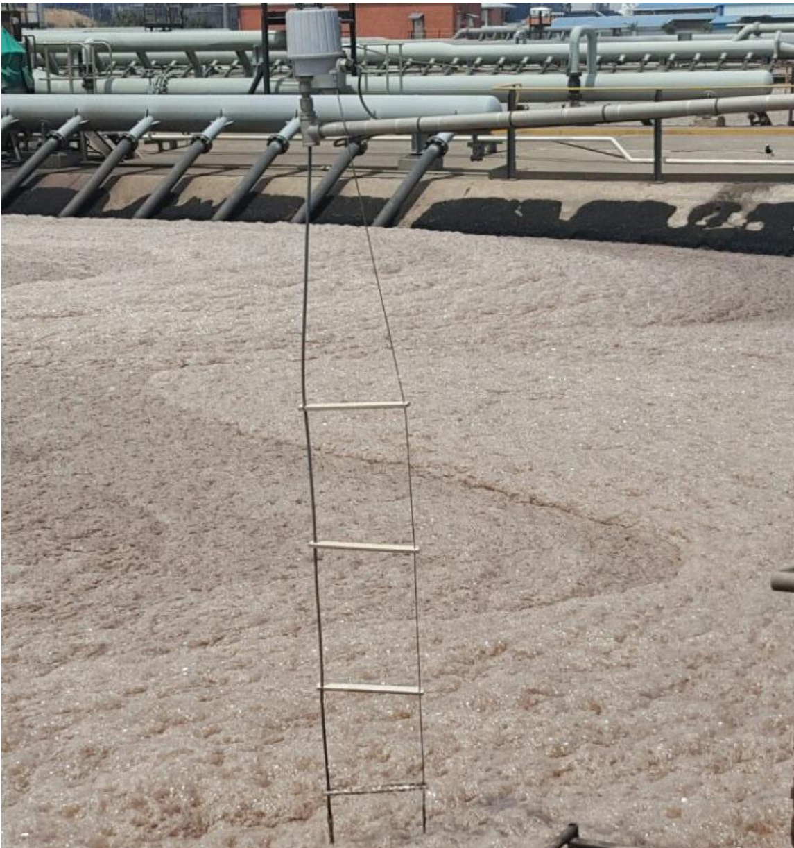
Figure 3.3: Foam height level probe in the bio-basin: foam height scenario (on site).
