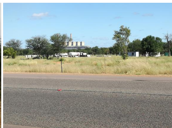
Photo 6: Site closed but bulk services incomplete
