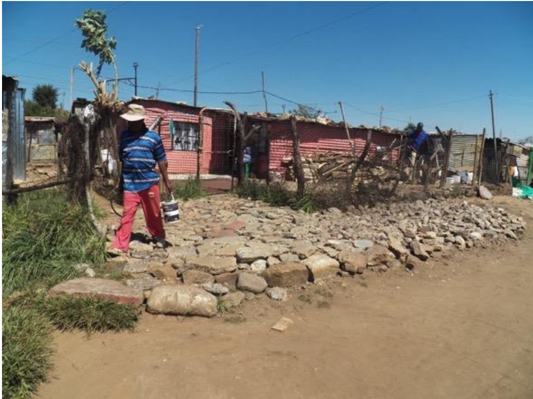
Figure 6.1: Rocks used for blocking water from entering the dwellings (also used for making the place less muddy after rains) (Source: Mpho Nenweli, March 2013) 18
