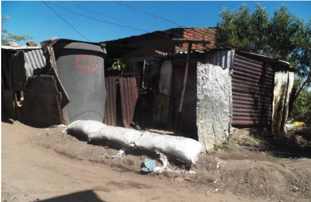
Figure 6.2: Sand bags being used to block water (Source: Mpho Nenweli, March 2013)
