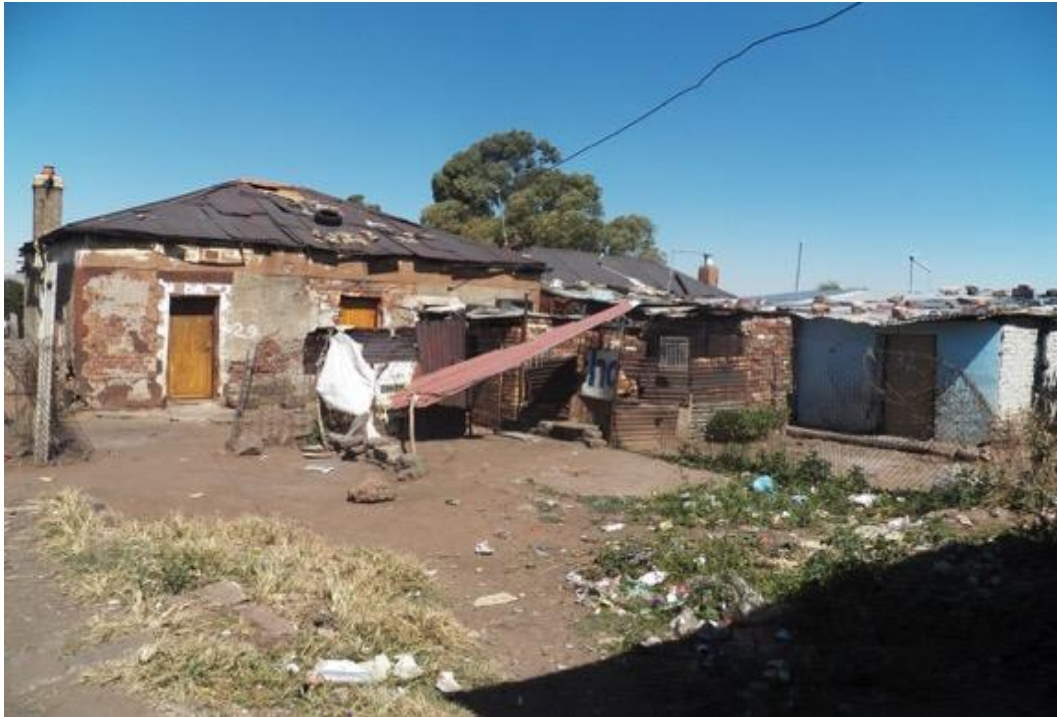
Figure 5.4: Rocks and other heavy objects to keep the roofs from collapsing due to strong winds and heavy rains in Freedom Charter (Source: Mpho Nenweli, March 2013)
