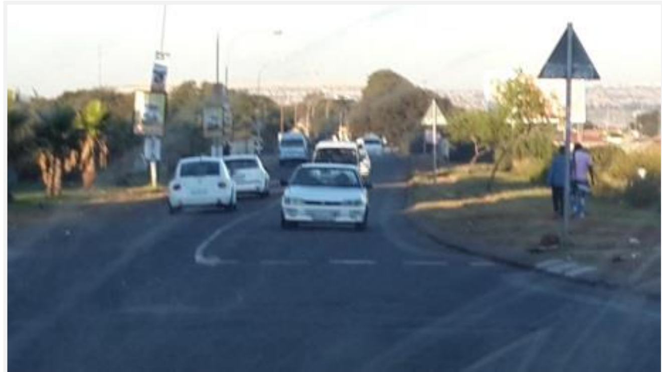
Fig. 15 Most of the road doesn't have any proper paved sidewalks and crossing zones for pedestrians. There are a number of trees but these are scattered all over the place
