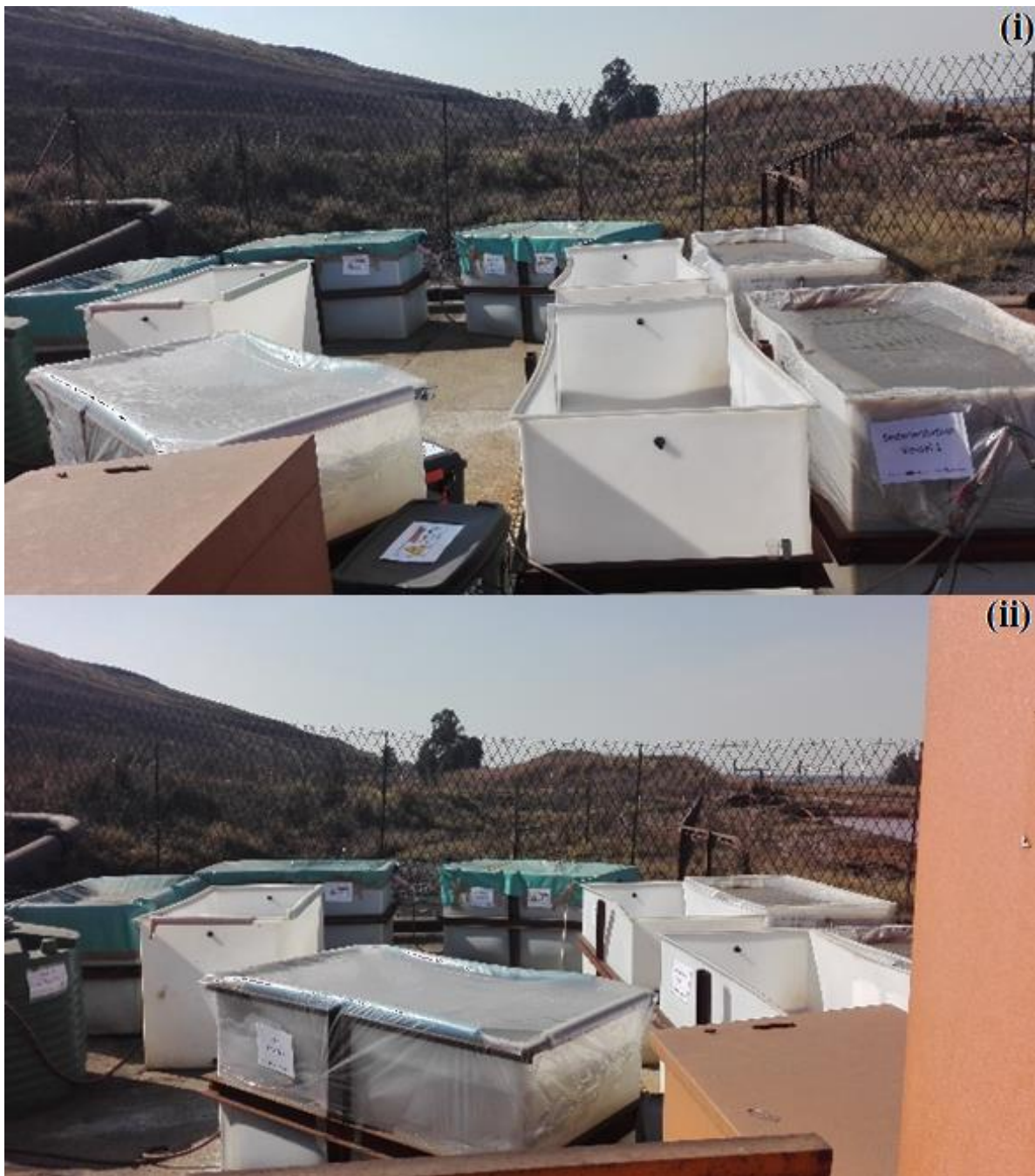
Figure 9-3: ((i) and (ii)) AMD remediation pilot plant at mine dam site
