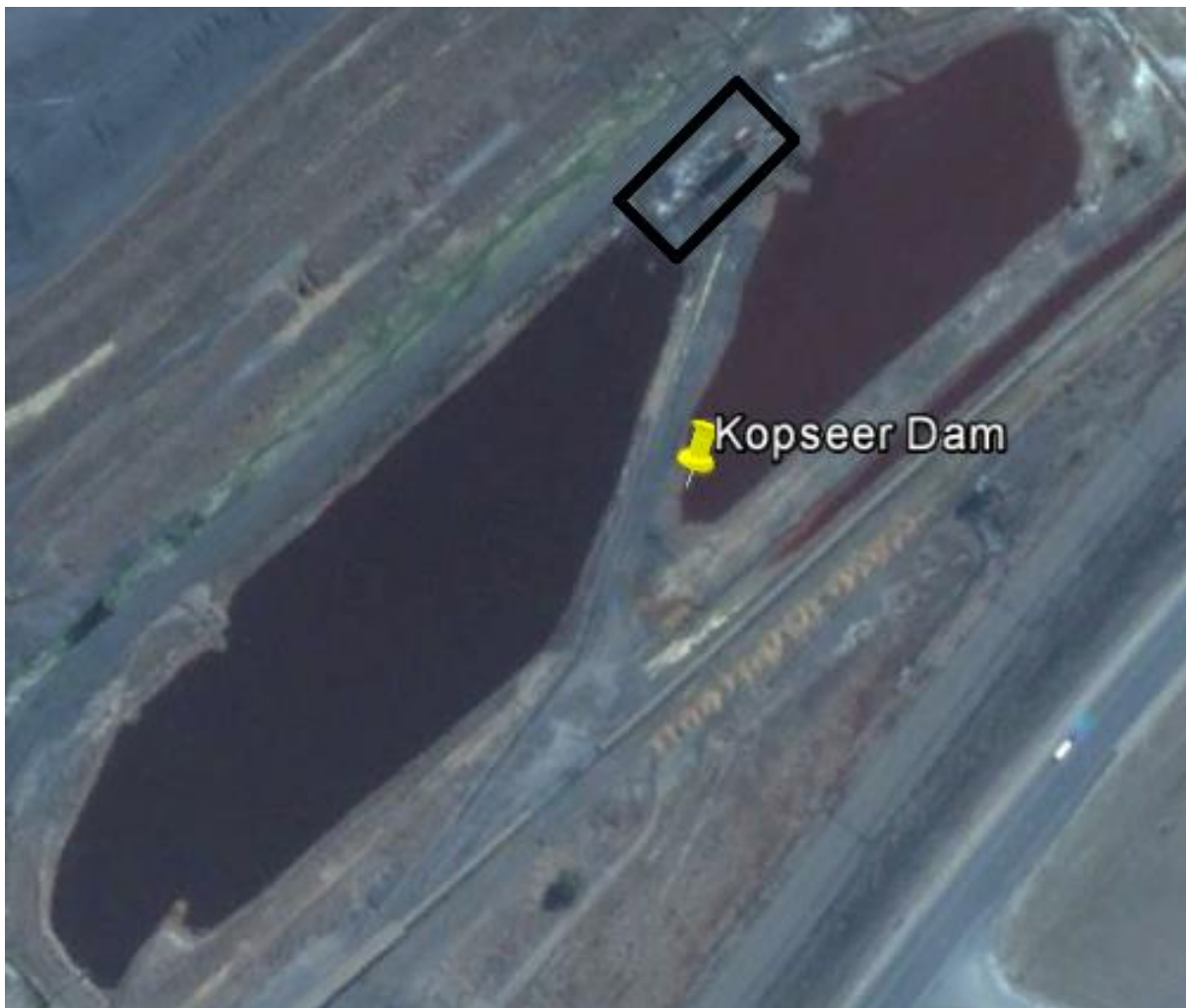
Figure 7-1: Top view of AMD tailings dam with area of construction outlined
