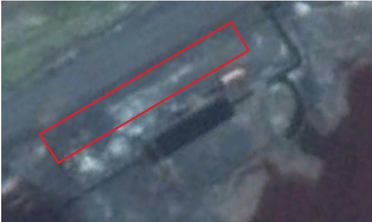
Figure 7-2: Top view of area to be used for construction of pilot plant at AMD tailings dam
