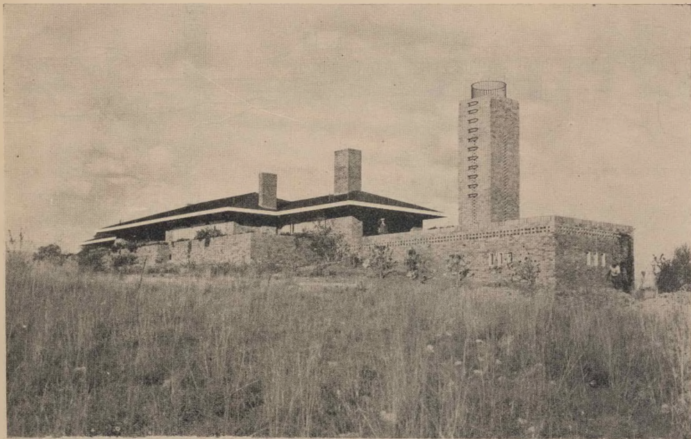
View from North-West from viewpoint 2 on the site plan, which gives a fine impression of the broad horizontal sweep of the house.
