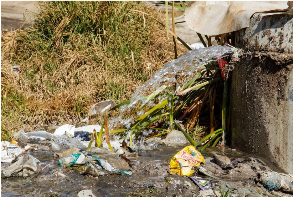
Figure 4.15 Sewerage leakage mixed with solid waste
